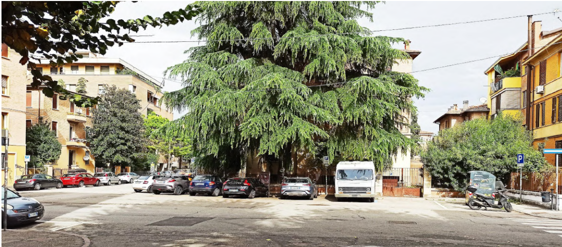
The area at the crossroads of Via Procaccini, Via Andrea da Faenza, and Via de Vincenzo before the intervention
